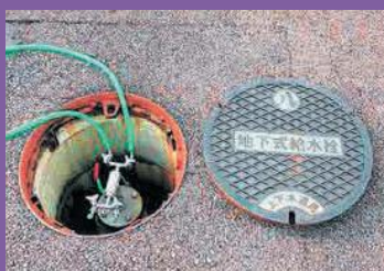
Underground hydrant (open the manhole cover to access the faucet)
