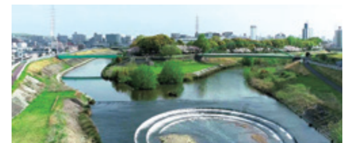
天白川と桶田川の合流点にある慶栄工 Construction designed for bed protection at the confluence of the Tempaku River and the Ueda River.
