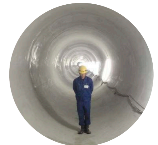
中村西部雨水調整池 Nakamuraiseibu Stormwater Storage Facility
