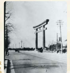
中村公園大鳥居完成 Completion of the Great Torii Gate at Nakamura Park
