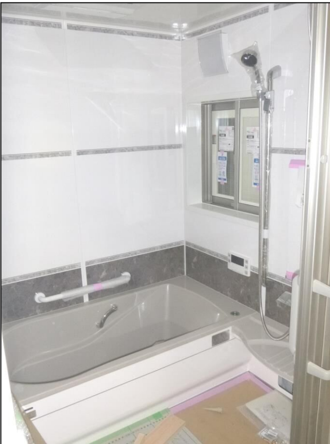
No. 11 壁① 1階 X7-Y10~11 仕上げ
