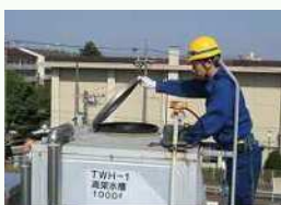
貯水槽の点検
