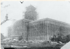
建築中の市役所本庁舎 City Hall Main Building under construction
